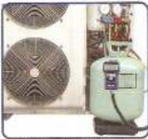
Charging for A/C System
