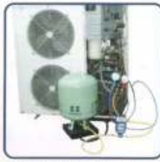
Charging for A/C system
